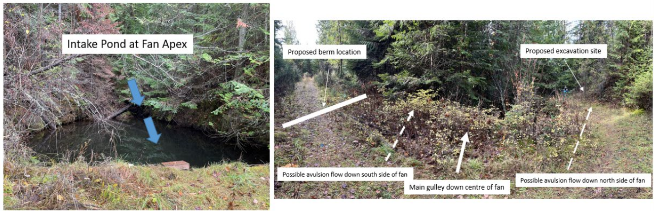
Photo 25. Water intake pond and road crossing at apex of McGregor Creek fan
