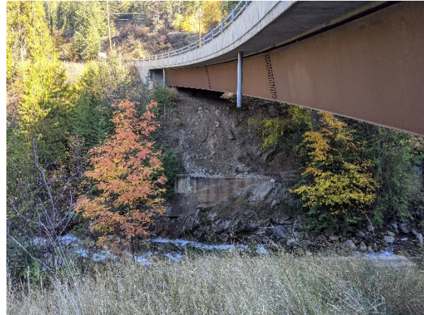
Photo 13. MoTI Highway 3A Bridge
