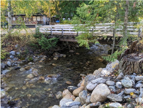
Photo 12. Local bridge across Akokli Creek on the fan
