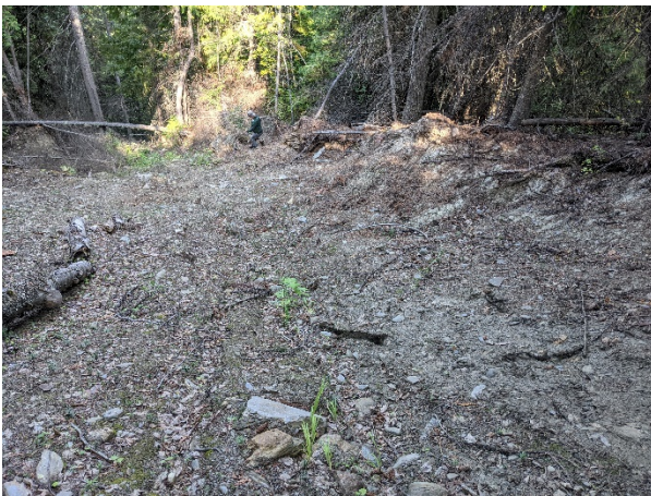
Photo 22. 5 km McGregor FSR landslide
