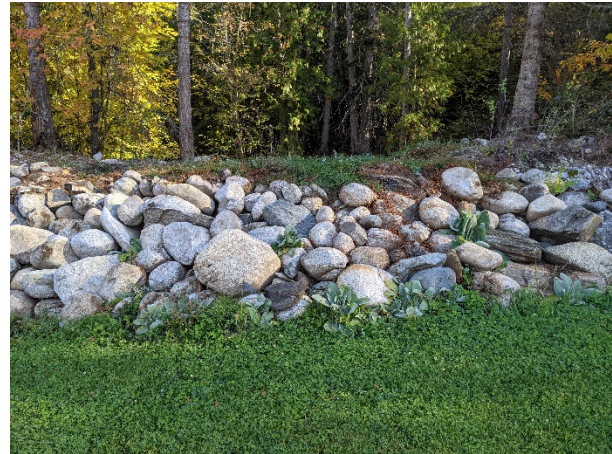
Photo 15. Berms constructed or reinforced on the Akokli Creek Fan
