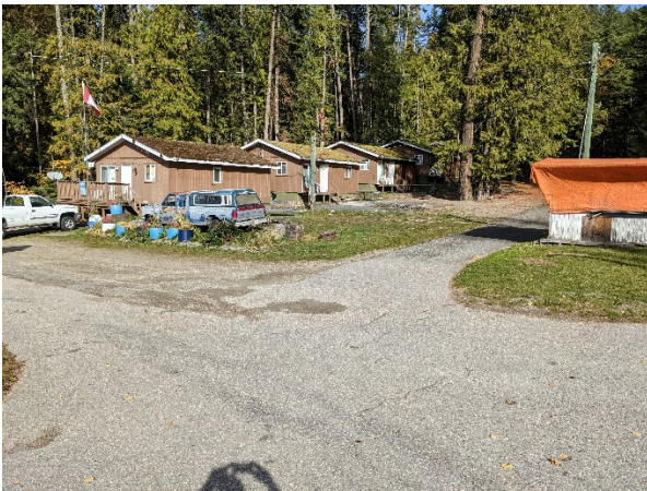
Photo 35. Cabins and office/dwelling on Lockhart Creek fan.
