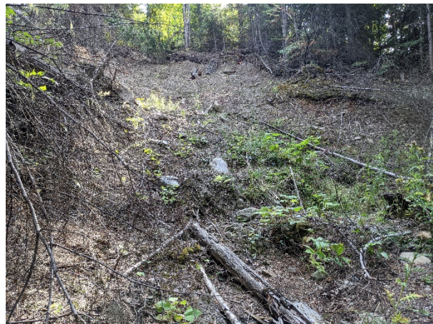
Photo 23. 5 km McGregor FSR landslide
