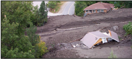
Figure 1. Debris flow material that was deposited on the Kuskanook Creek fan after a rainfall event in August 2004.
