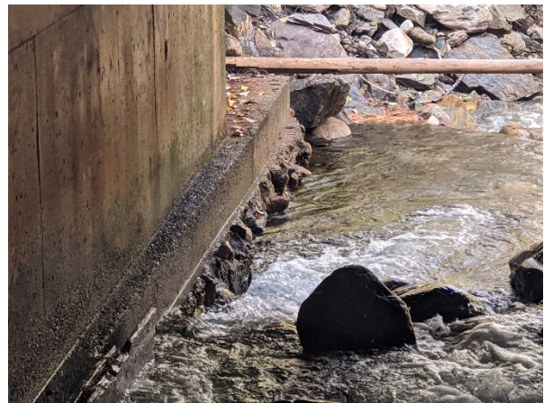
Photo 32. MoTI bridge over Lockhart Creek
