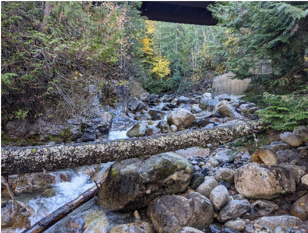
Photo 14. Akokli Creek Channel below MoTI Highway 3A Bridge
