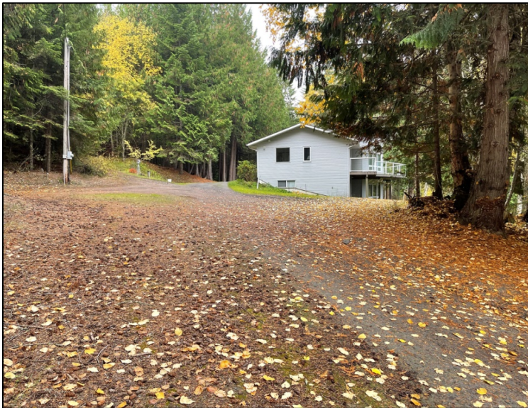
Photo 30. View looking south at house at 12850 Hwy 3A. The fan slopes left to right. The house is 240 m from the apex of the North Mack Creek fan.
